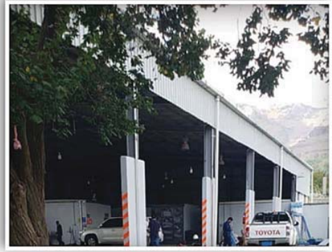
Construction of Maintenance workshop Client : Yemen motors company
