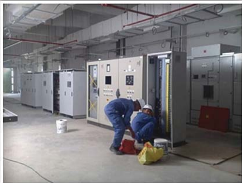
Electrical construction works Client : Tanmia for oilfield services
